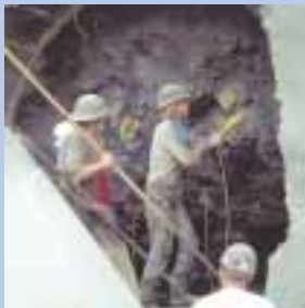
Tunnelers set dynamite for Exploratory Tunnel.
