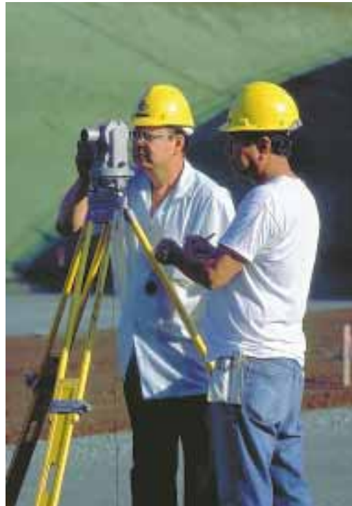
Surveyors set alignment for H-3.
